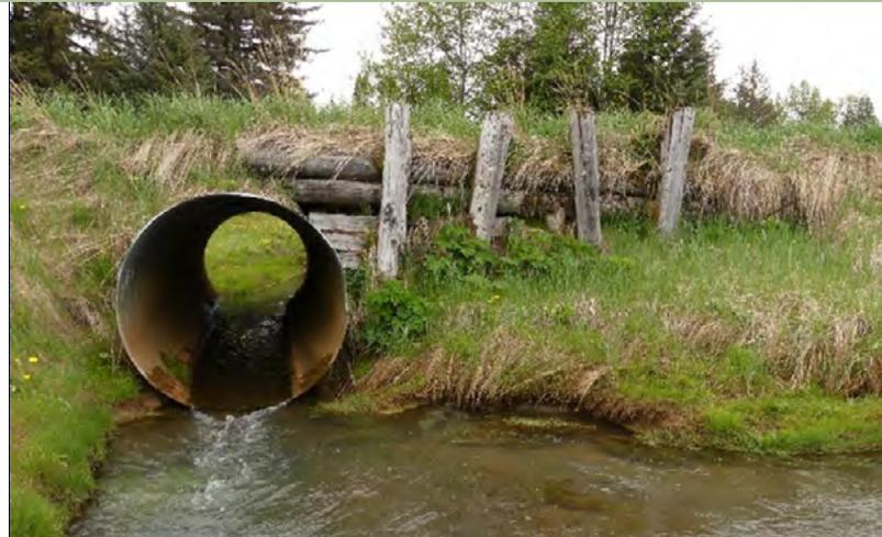
According to the FWS, this too-small culvert perched above a creek is impeding 6 miles of rearing habitat for juvenile coho salmon in Gustavus, Alaska. This creek is also used by Dolly Varden and cutthroat trout. Through IJA funding, this culvert will be replaced with a timber bridge.
