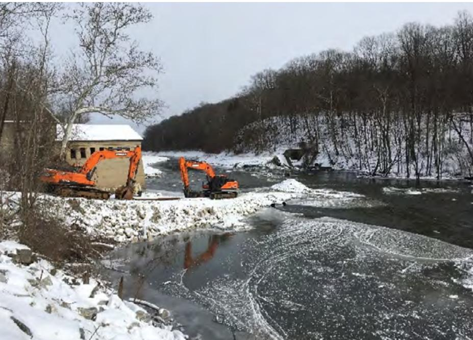
Funding from the Delaware Watershed Conservation Fund went to a nonprofit to remove the Columbia Dam in Knowlton Township, New Jersey. The dam was originally constructed for ice harvesting and to supply power, but it also stopped American shad from reaching spawning grounds. According to New Jersey Fish and Wildlife, within 6 months of the last portion of the dam being removed, American shad were seen upstream of the dam for the first time in more than 110 years.
