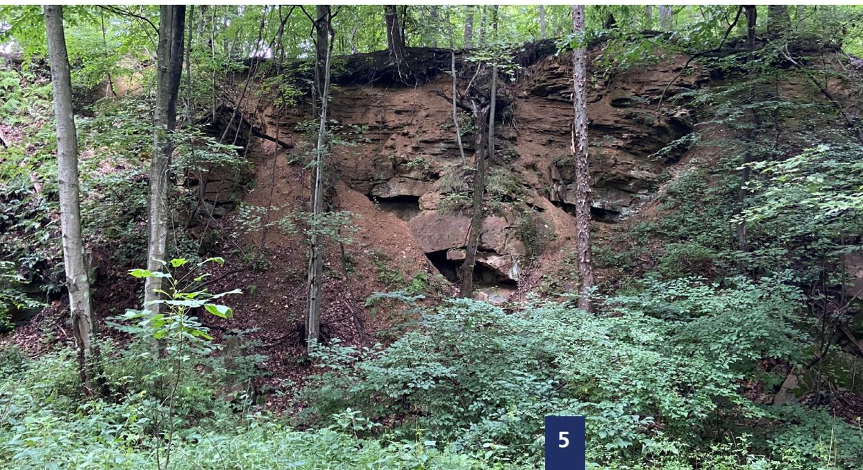
Highwall and collapsed entrances in Morgantown, WV. This site includes approximately 4,725 linear feet of highwall ranging in height from 15 to 40 feet, 13 open entrances, at least 10 collapsed entrances, and approximately 2,100 feet of clogged stream.
