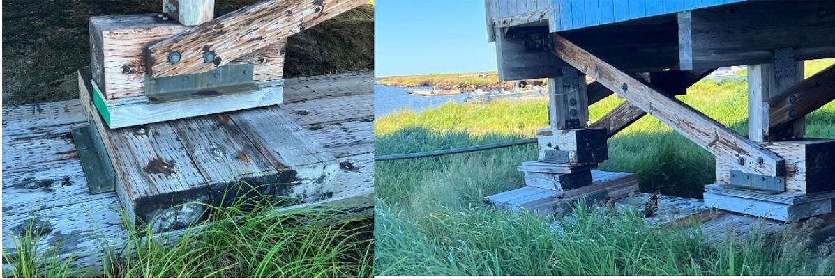
This foundation is unstable due to permafrost degradation. Blocks are placed under the original foundation to help stabilize the structure.
