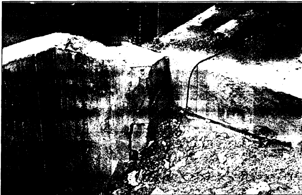
Figure 6. Close-up of cracks in the wing wall adjoining the bridge shown in Figure 5. (Office of Inspector General photograph)
